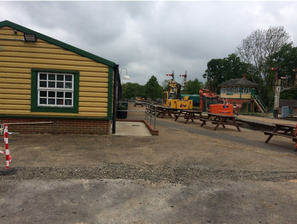
View towards Carriage sheds
