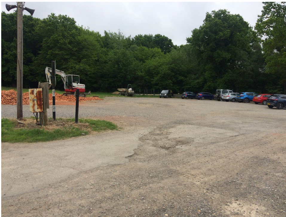
Reverse view of car park
