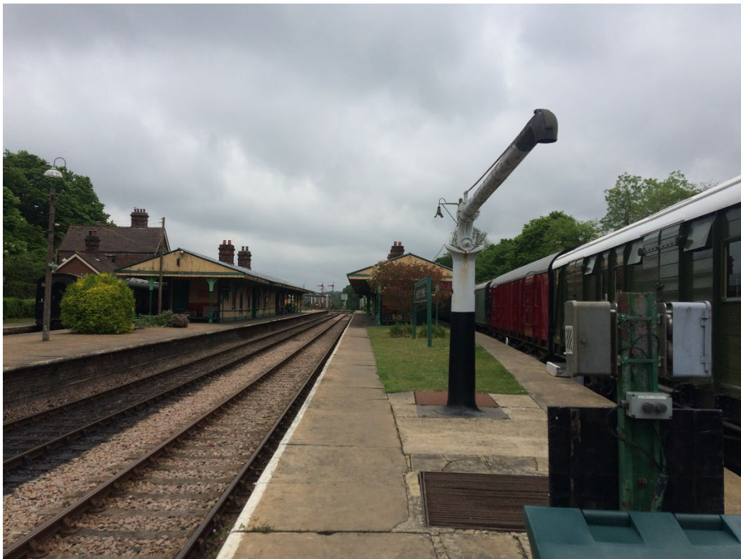
Further view platform area
