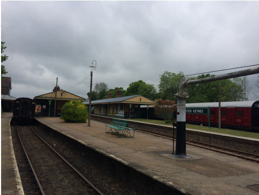
Further view Platform area
